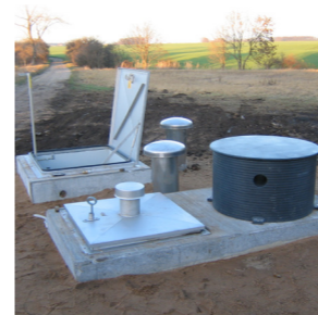
Exterior view of the pumping station
