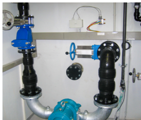
Retrofitting with a vortex impeller pump for increasing the flow rate
