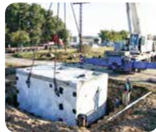
Installation of a pump station - all from one source
